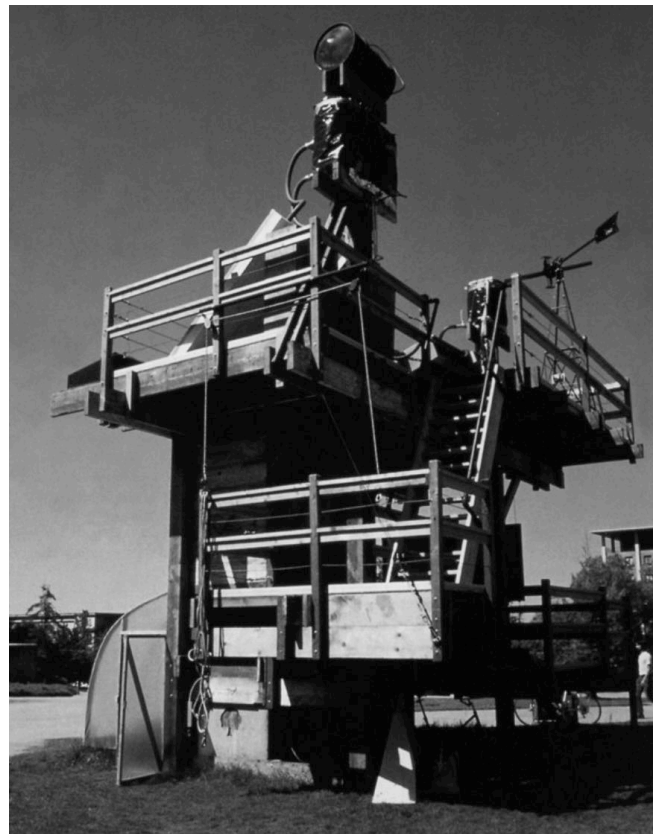
Figure 9. Energy pavillon Berkeley, 1973
